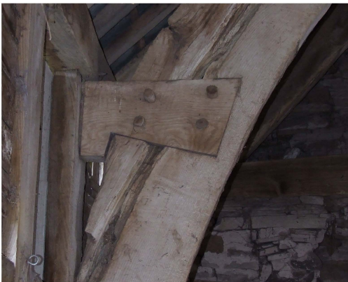
Above: original wattle panel intact in north wall Below: detail of sixteenth century carpentry on eastern cruck-truss.
