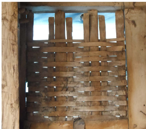
Above: original wattle panel intact in north wall Below: detail of sixteenth century carpentry on eastern cruck-truss.
