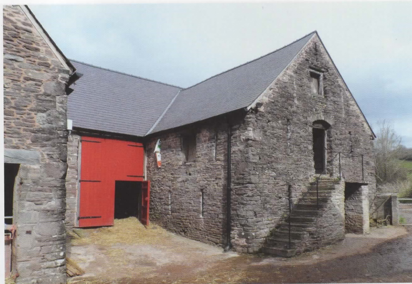
TOP: Barn at Great Trerhew Farm, Llanvetherine, Monmouthshire, after restoration.
