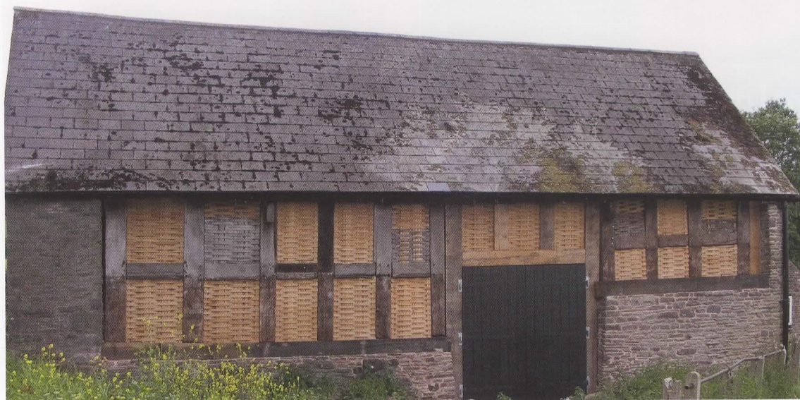
TOP: Croft Barn, Whitecastle, Monmouthshire, exterior after restoration. The barn was originally part of the Great Trerhew estate.
